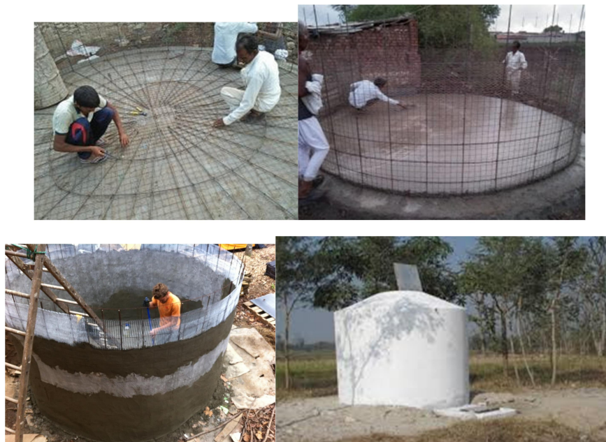
FIGURE:- FERRO CEMENT TANK
