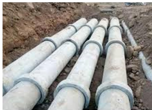
FIGURE:- COLLAR JOINT
