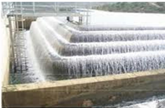
FIGURE: CASCADE AERATOR
